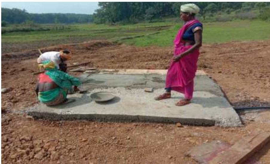
Construction of sump in Serajhar village Dindori by the community
